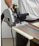
• Cut the panels to fit (Hand saw with set beam or circular saw with rail).
