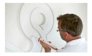
Retouchal of the wall and ceiling joints as well as the mitres with ADEFIX® adhesive (see GLUE CONSUMPTION).
