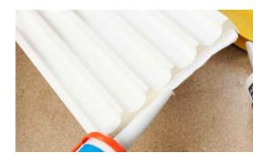
• Glue the vertical and mitre joints with ADEFIX® PLUS joint adhesive (see GLUE CONSUMPTION).
