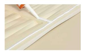
Apply a continuous line (bead) of ADEFIX® PLUS mounting adhesive to the rear mounting surfaces (see GLUE CONSUMPTION).
