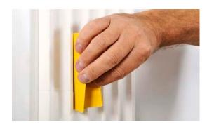
Allow the glue to dry (min. 6 hours) then sand the outsides of the joints lightly (sandpaper 150 grit or less) and retouch them again with ADEFIX® adhesive.
