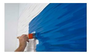
• If final painting has not been undertaken before assembly, apply the final coat of paint to the panels after drying (approx. 6 hours) and within 4 weeks (see FINISH).
